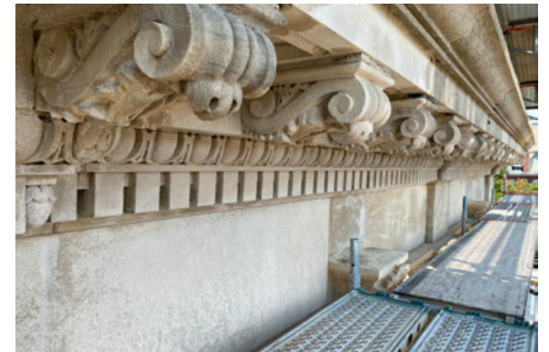
CLEANING & RESTORATION PROCESS
